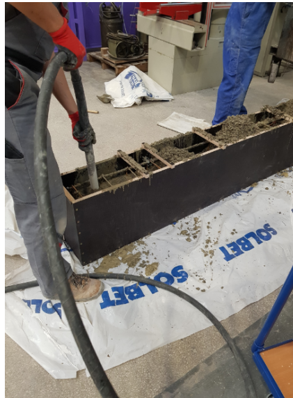
Figure 6.10: Vibration during pouring the concrete and collecting of specimens
