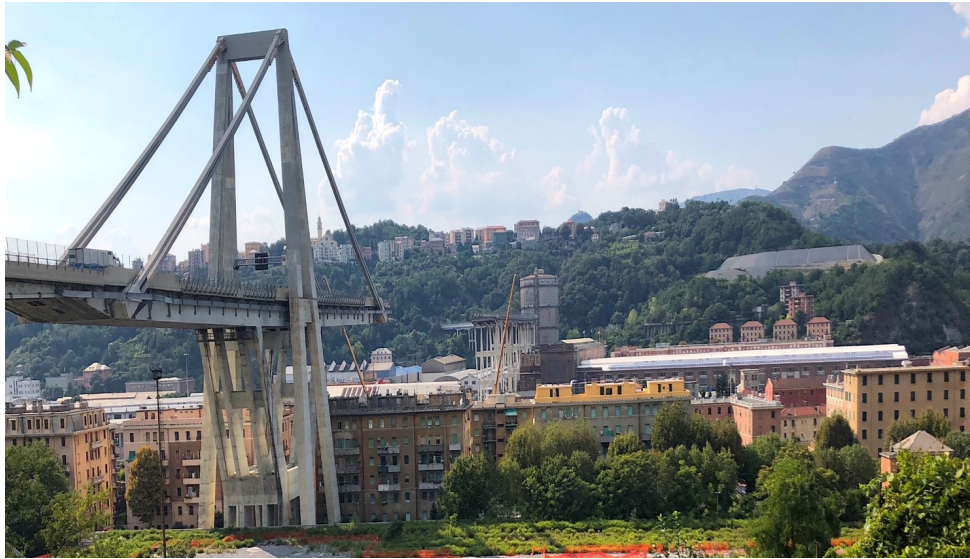
Figure 1.1: Photo of Morandi Bridge after the collapse (Ferraris, 2018)
