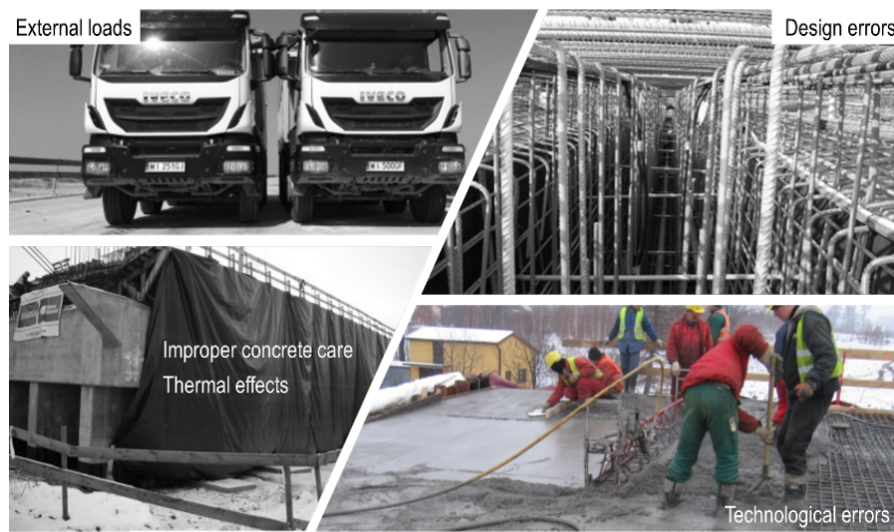
Figure 2.12: Causes of concrete cracking
