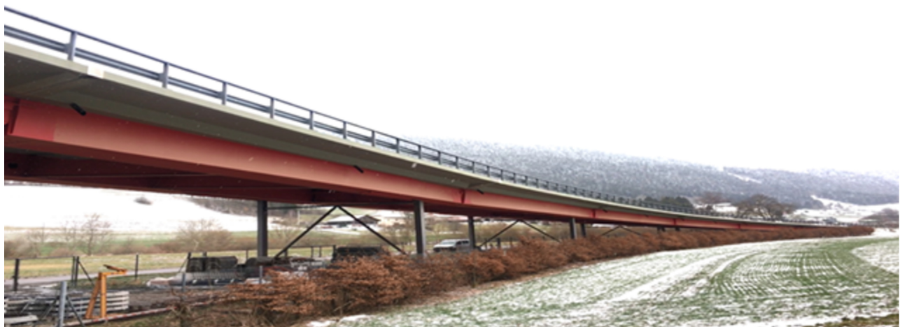
Figure 1. View of the investigated steel-concrete composite viaduct
